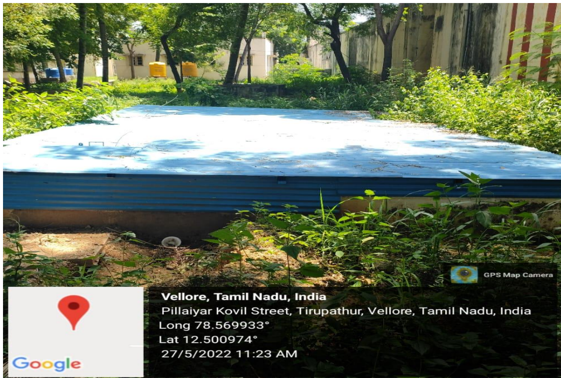
Filtration and purification of liquid waste water from Rinaldi hostel
